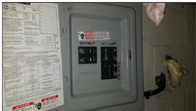
7.1 Siemens Subpanel in Crawlspace
